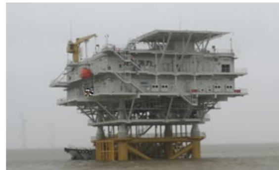
Jiangjiasha Offshore Booster Station.
