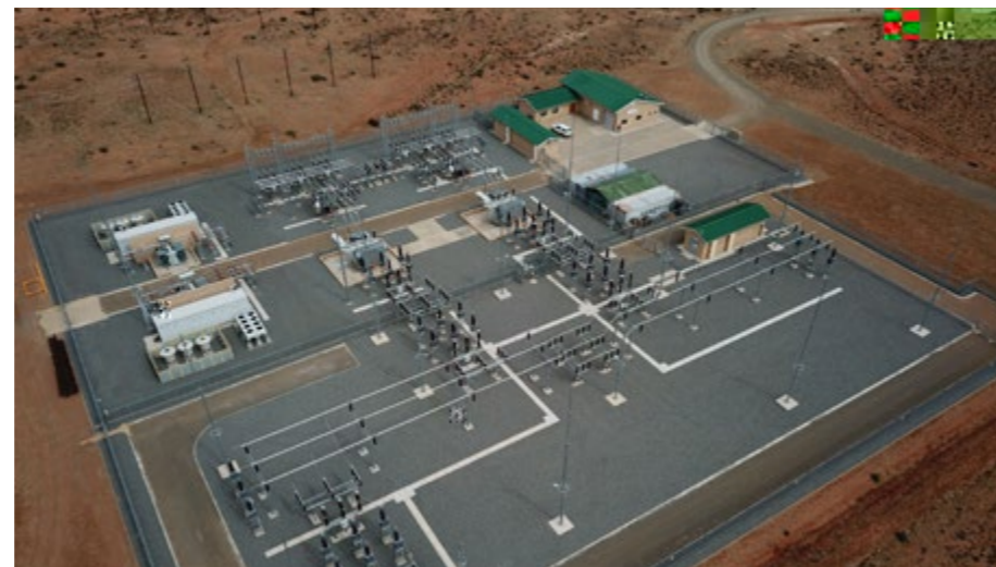
All electric transmission and transformation equipment are procured locally, increasing job opportunities for equipment manufacturers and local community.
