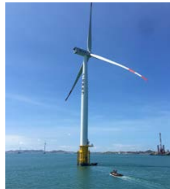
Longyuan Fujian Company's offshore wind farm staff sails to work
