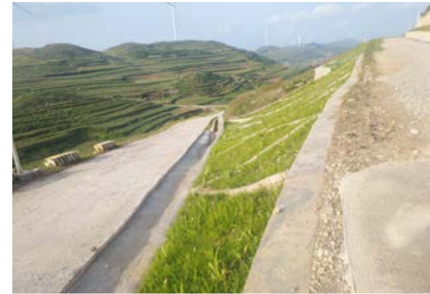
Longyuan Guizhou Company Weining Xiaohai Wind Power Project implemented the principle tht water and soil conservation construction designs, constructs and puts into operation with the major engineering construction. The picture shows the water and soil conservation governance achievement demonstration.
